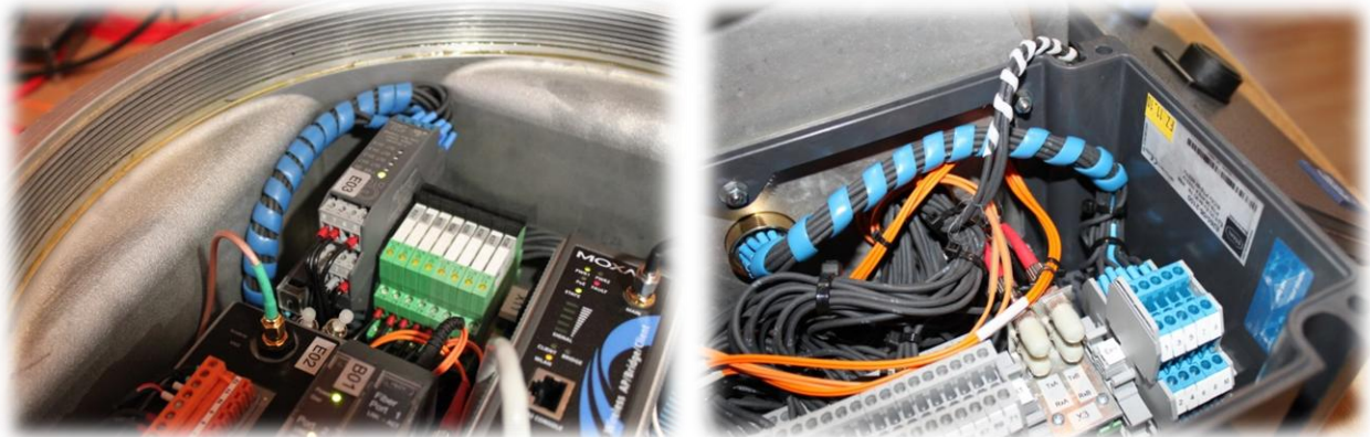
Fig.8.2: Intrinsically safe circuits of the ExConnection Rail
