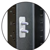
Ground Studs located directly on rack channel
