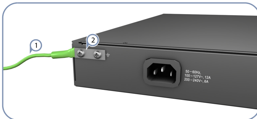
① Grounding Wire
